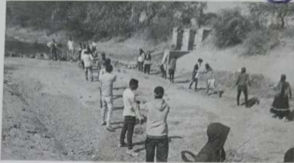
Road Construction by student's year 2018-19
